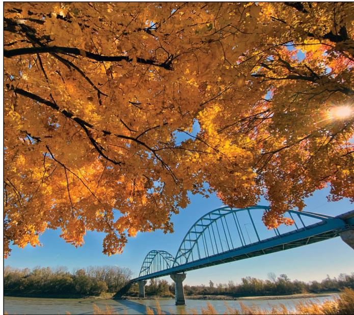
View of the Missouri River and Centennial Bridge from the shelter at Riverfront Park in early November.
