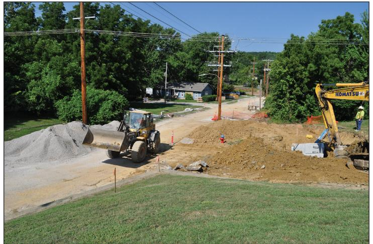
**Thornton Street:** This \$5 million project continued throughout the pandemic. It is still on schedule to be completed by the end of 2020. Work in the summer and fall included a reinforced concrete box culvert near the Municipal Service Center, tearing out existing street and roadbed from 10th Avenue to Maple Street and placing aggregate base for the street. The final layer of asphalt will be placed over the entire project, from 10th Avenue to South Fifth Street.
