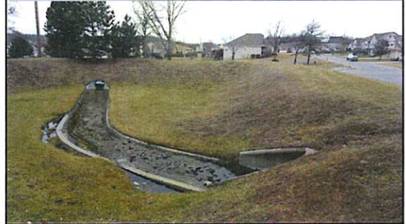
This Basin Has A Concrete Trickle Channel
