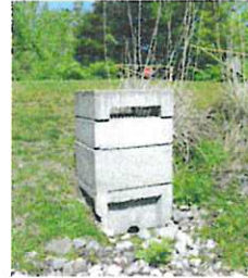
Basin Outlet Structure
