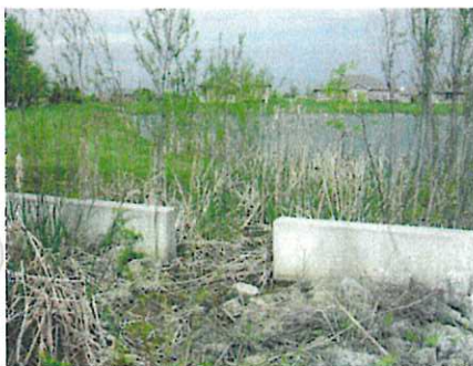
Detention basin overflow weir
