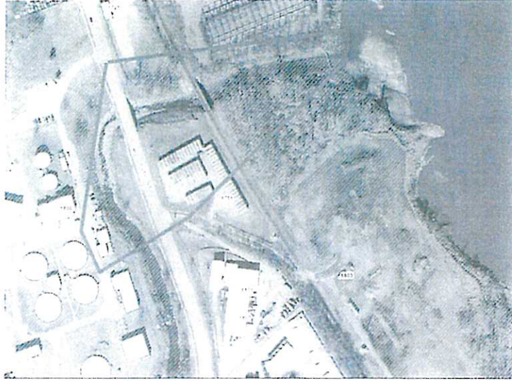
Aerial View of Wastewater Treatment Plant
