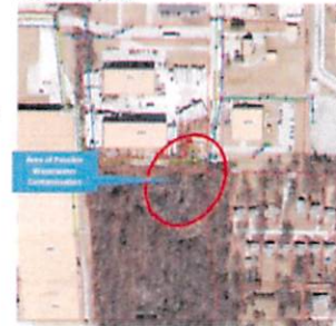
4808 Brewer Place Sewer Overflow November 13, 2020
