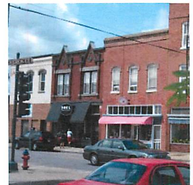
Preservation of historic and contributing structures should be pursued in the West Gateway. New and infill development should be context-sensitive and contribute to the overall sense of a vibrant, active environment.
