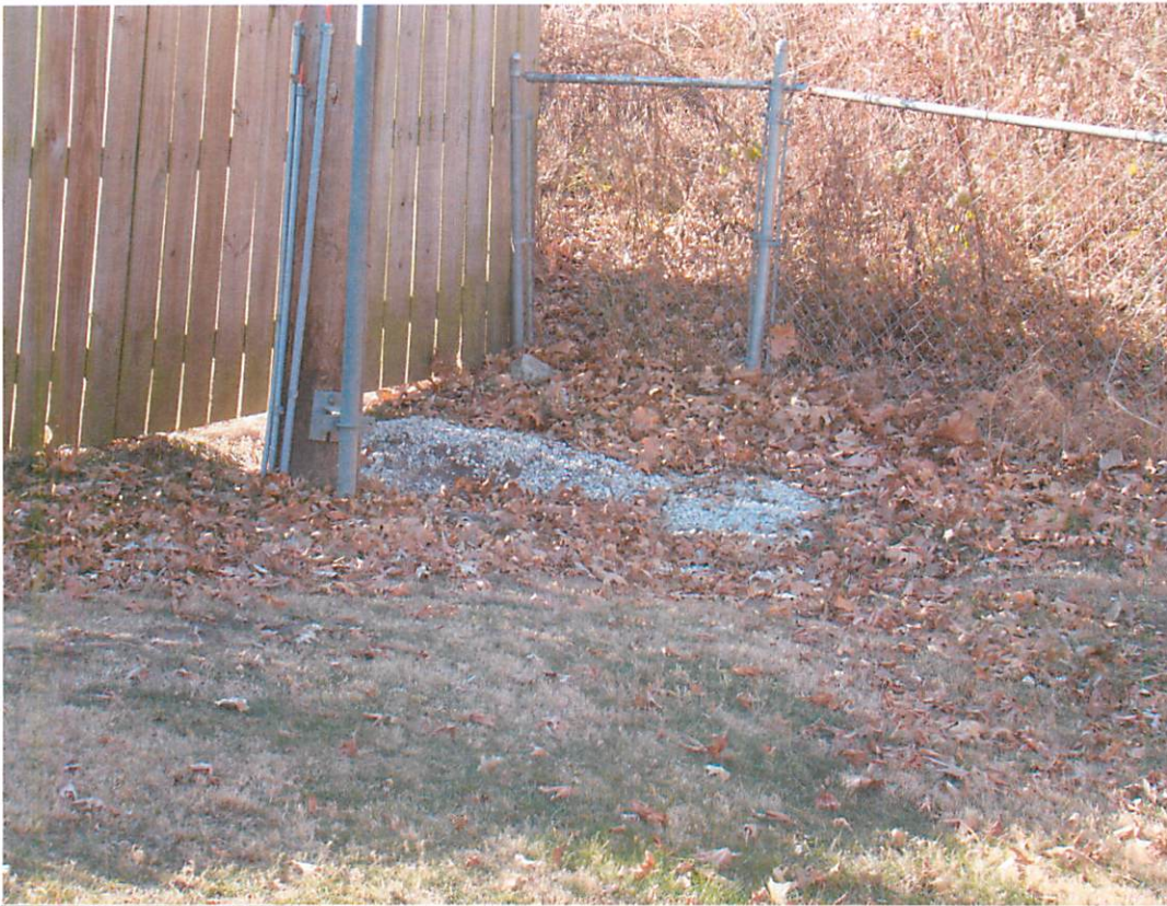
#3: The Southwest corner of 1106 South 14th St. Water from the woods and neighboring yards directly south enters this portion of the yard
