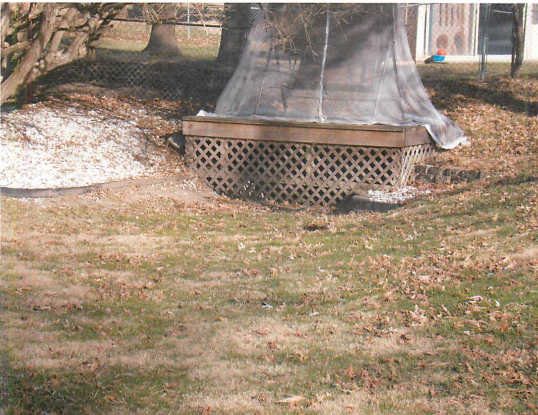
#4: The water from the woods and neighboring homes flows into this area of the back yard of 1106 South 14th Street and is diverted directly into this storm water run off tube.
