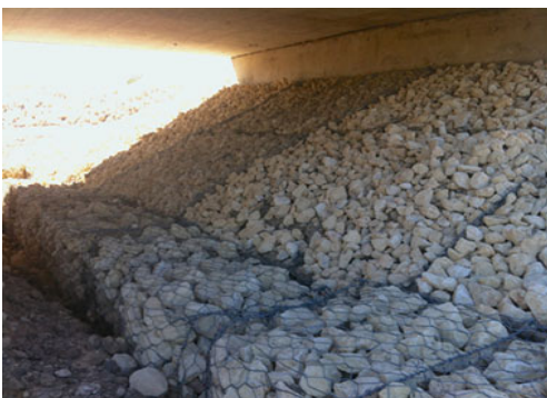
The City places riprap under bridges to protect the structure from erosion
