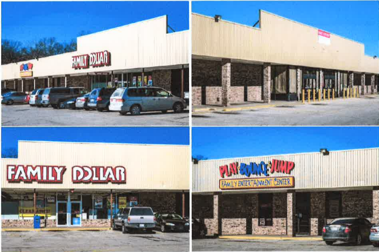
Figure 1: Sampling of Conditions
