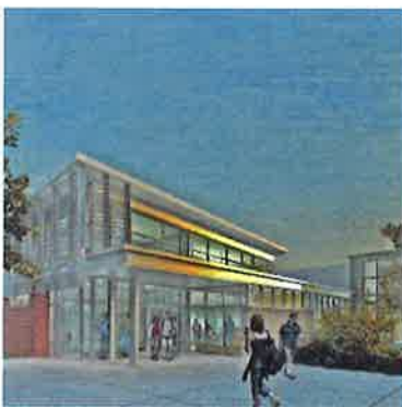
Substantial building forms at Metropolitan Avenue and 4th Street is envisioned by the master plan to present a significant visual experience into Leavenworth and the character areas of Downtown.
