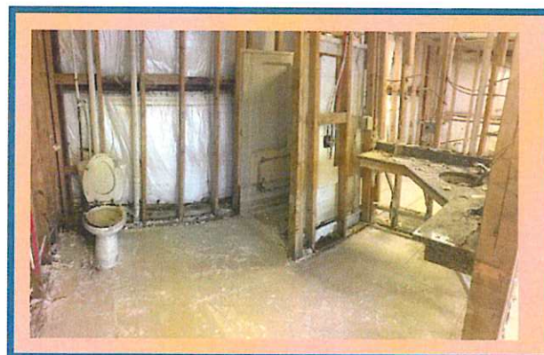
Restroom with Damaged Infrastructure Removed - April 2019
