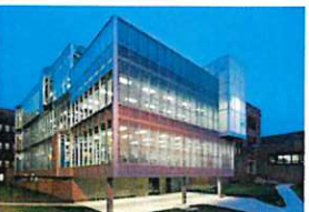
OPS North High School Science & Technology Addition
