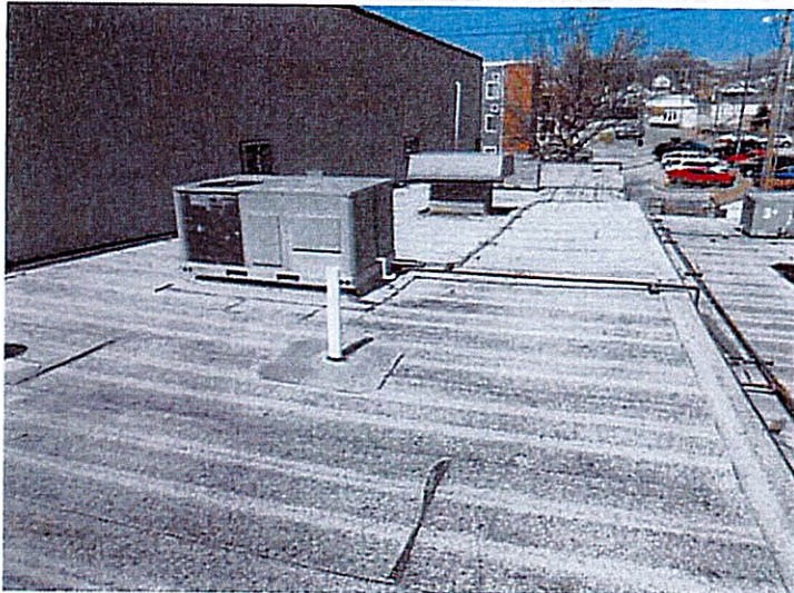
26. Looking north over the western half of the roof.
