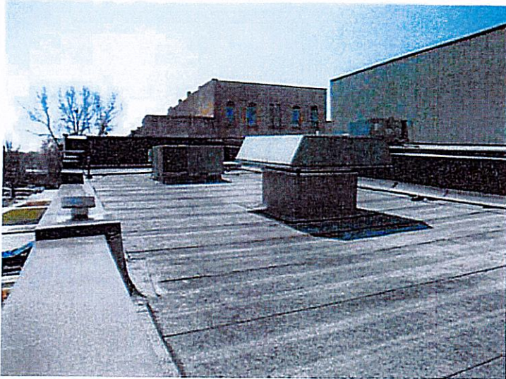
23. Looking south at the roofing on the east half of the building.
