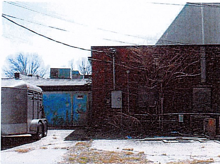
4. Building as seen from the northwest. The brick is the western half, and the blue finish is the eastern half.
