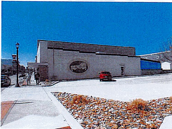
2. East/right side of building.
