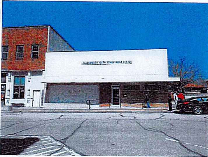
1. Front/south side of building.
