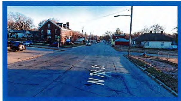
Pre-Construction of N. 7 th Street
