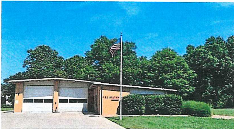
Fire Station #3 was built in 1965. At the time, ADA and separate gender facilities were not considered. Additionally, the facility continue to experience drainage and sewer problems.
