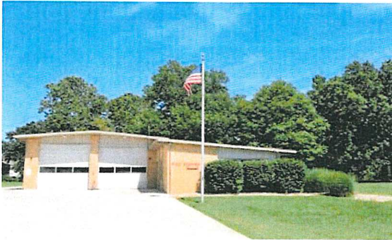
Fire Station #3 was built in 1965. At the time, ADA and separate gender facilities were not considered. Additionally, the facility continues to experience drainage and sewer problems.
