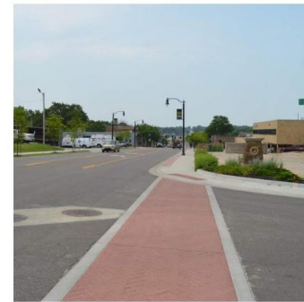
COLORED CONCRETE CROSSWALKS
