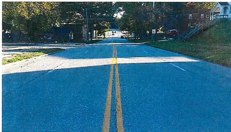
Segment #6 – Looking south at Kickapoo Street
