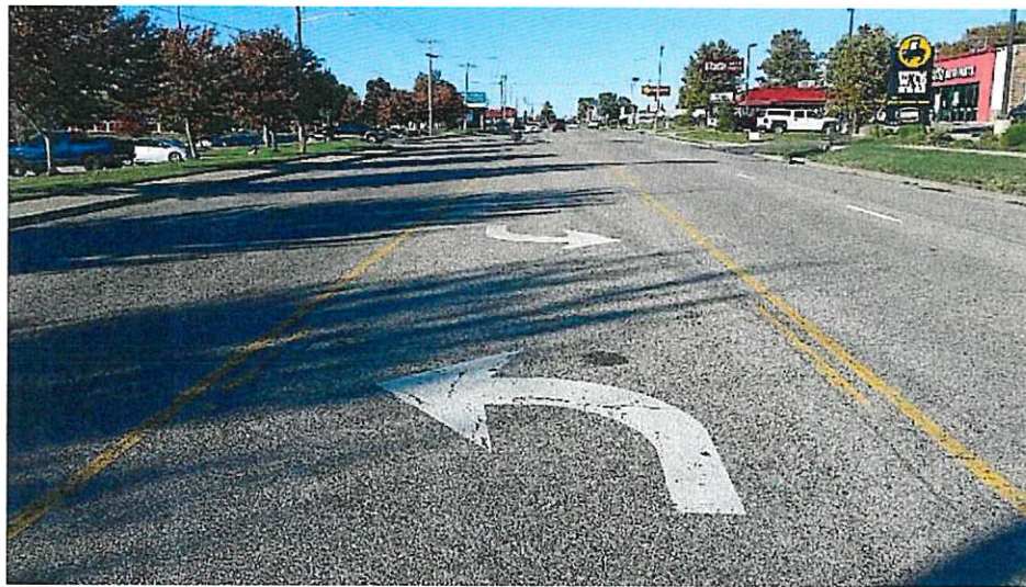
Segment #1 – Looking north from 700' north of Eisenhower Road
