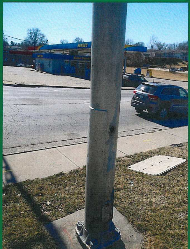
Welded Repair to Reinforce Pole
