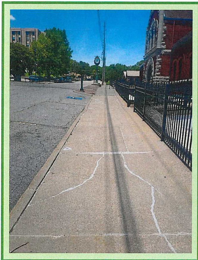
Failed sidewalk ramps and crosswalks at Delaware & Esplanade (Riverfront Community Center)
