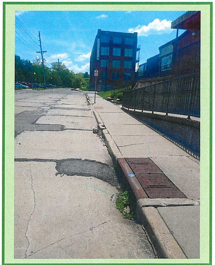
Failed sidewalk ramps and crosswalks at Delaware & Esplanade (Riverfront Community Center)
