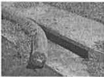
Curb Inlet Filter.
