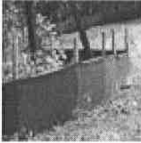
Silt Fence Silt Fence controls sediment runoff from construction sites where the soil has been disturbed.
